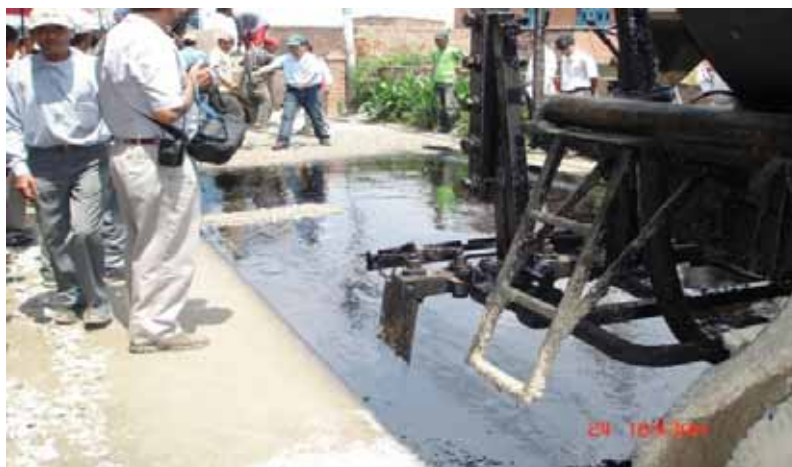
Photograph 5. Aggregates being sprayed by hand over the freshly sprayed binder by distributor
