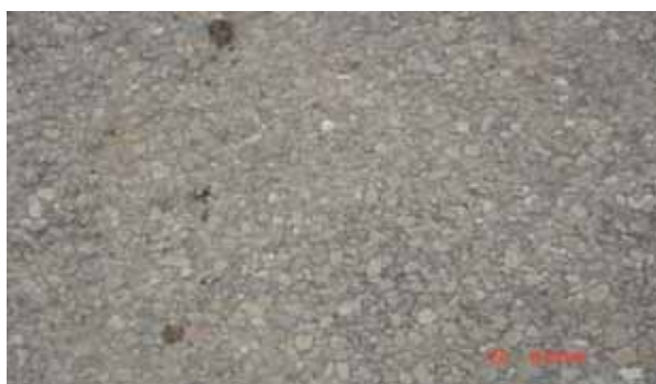
Photograph 8. Finished Single Otta seal surface seen after the opening of traffic over the base course
