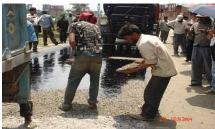
Photograph 5. Aggregates being sprayed by hand over the freshly sprayed binder by distributor
