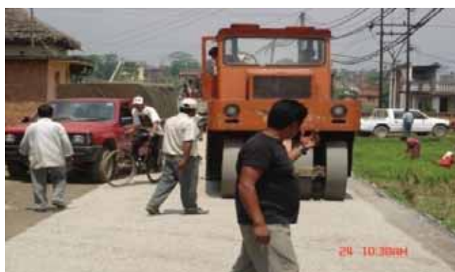
Photograph 8. Finished Single Otta seal surface seen after the opening of traffic over the base course
