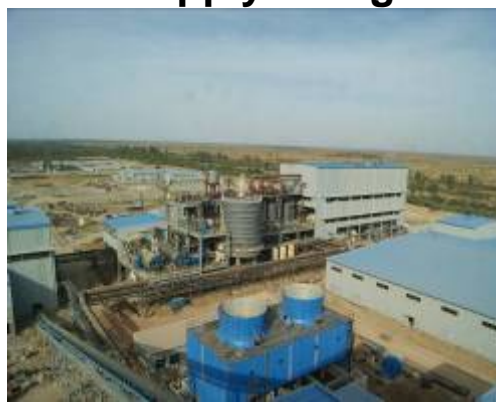
Sugar plant in Mali
