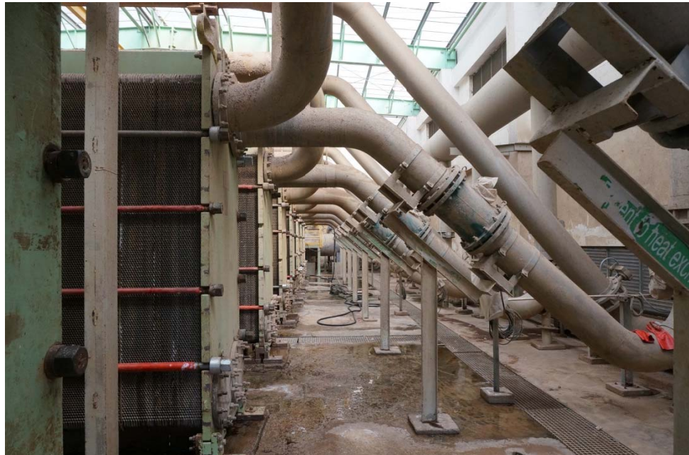
Figure 2: Plate heat exchangers in Asia Symbol Pulp and Paper factory in Rizhao
