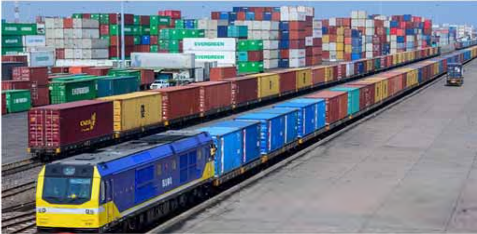
Double track projects: 7 lines (993 km)
