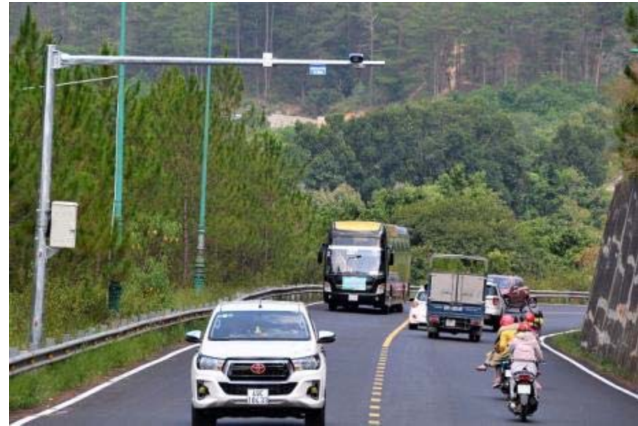
Traffic camera installation on NH 20 26 April 2019
