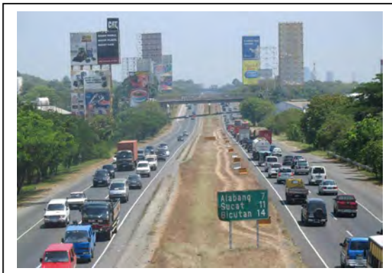
Asian Highway (AH26) South Luzon Expressway Extension Project
